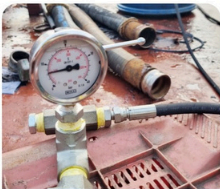
Pressure test process
