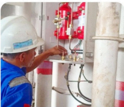
Time delay of CO2 system
