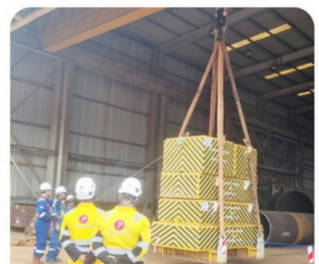
Load test OH Crane
