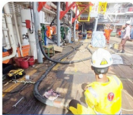
Pressure test oil hose
