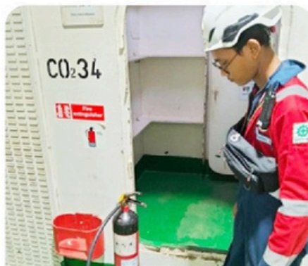
Inspection of Fire Extinguisher
