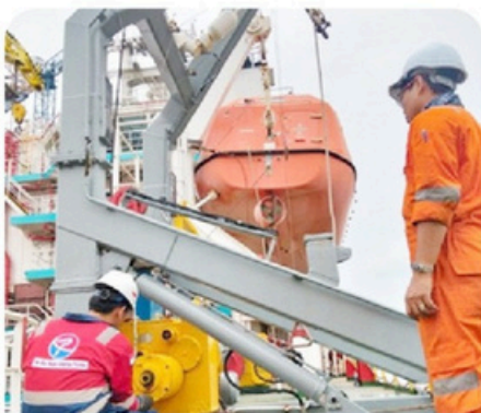
Replace wire of Lifeboat
