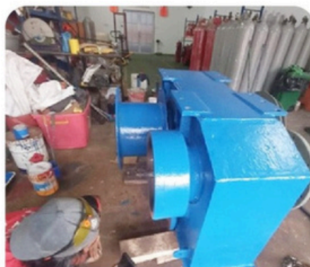
Overhaul of winch system
