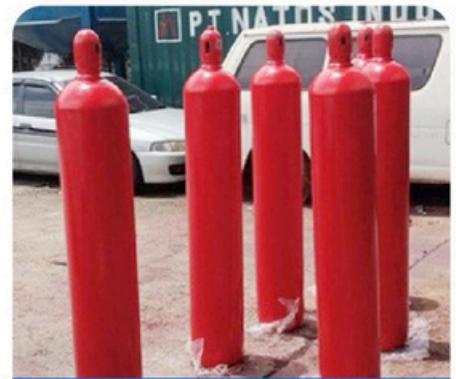
Repainting CO2 System
